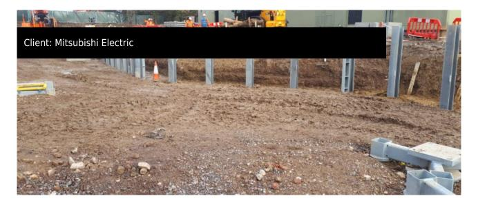
80 Galvanised Posts to 8m installed within 4 days @ 1.5m spacings. 6.5m post embedment, 1.5m of post AGL.
