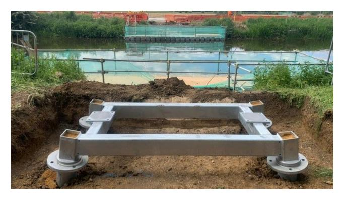
ScrewFast's site team were on site this week and completed the installation of 8 helical piles with 2 Grillages to support a footbridge in Elton, Cambridgeshire.
