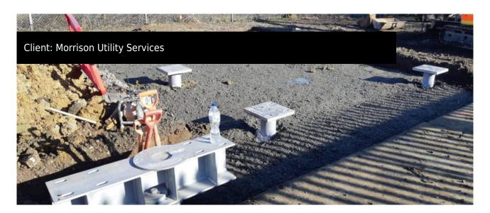
As part of ScrewFast Foundations long-standing relationship with Morrisons Utilities, we were contracted to install foundations at two further locations. The ScrewFast design team recommend helical pile foundations at the majority of substation sites because the installation process requires minimal plant and no excavation. This significantly reduces risk involved with the foundations process with the proximity to overhead high voltage cables, as well as underground cables and services.
