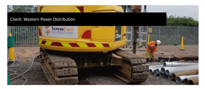
Working for client Western Power, ScrewFast carried out the installation of 45 No. Helical Piles for Ross-on-Wye Substation. The foundations were installed, ready for loading in just 10 day shifts.
