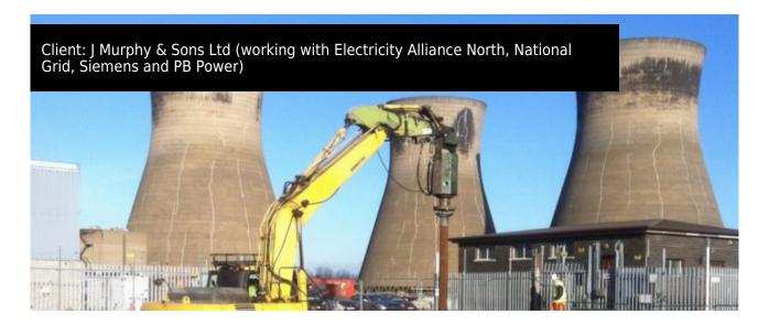
Brief: Design and Install helical piles solution as a cost effective alternative to concrete.
